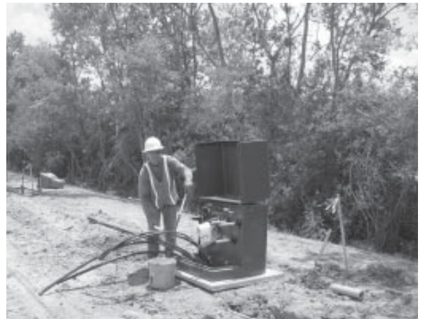
Fig. 6 Contractor completing installation of JSRP Transformer
