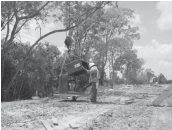
Fig. 5 Contractor feeding cable through compartment
