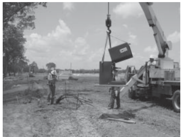
Fig. 4 JSRP Transformer descending to final installation site
