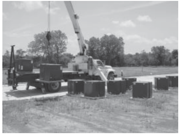
Fig. 2 Boom truck crane operator off-loading JSRP Transformer
