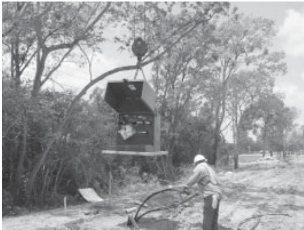
Fig. 3 Contractor setting up for installation
